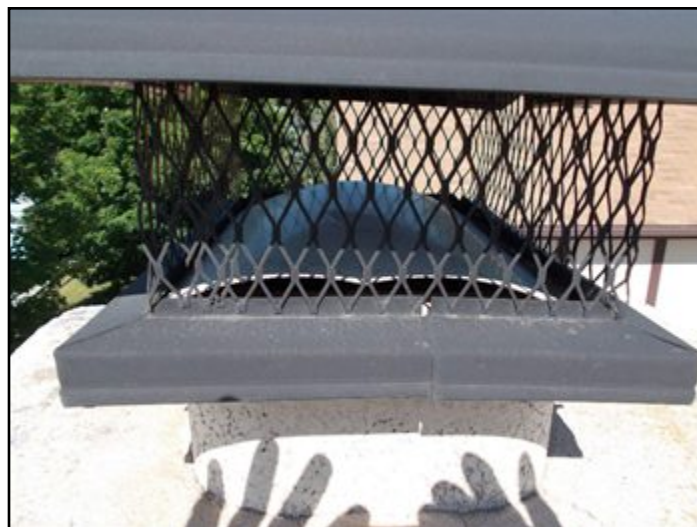
32. remove obstruction at chimney top
